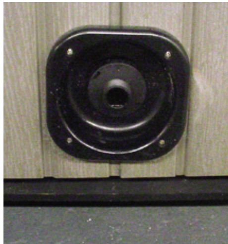
Figure 20. Cabinet mounted drain valve
