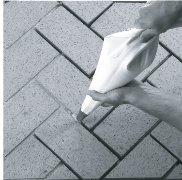
Figure 20 - Grouting Brick
