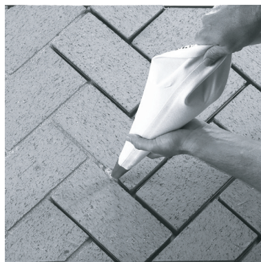
Figure 25 - Grouting Brick
