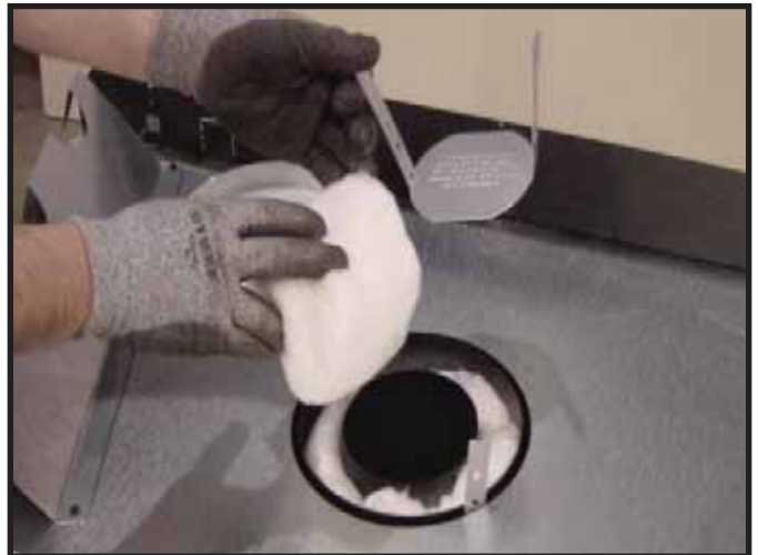
Figure 9.5 Remove the insulation basket and white insulation from the center vent pipe.
