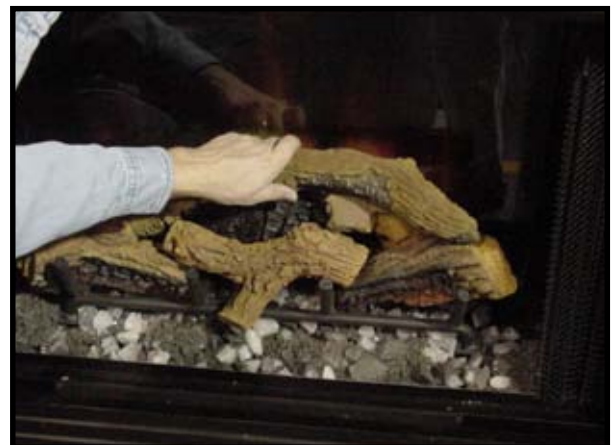
Figure 11 - Replacing Log Assembly
