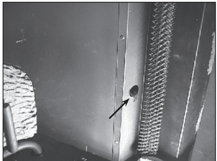
Figure 7.1 Outside Air Kit Handle Location
